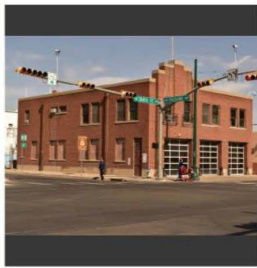
ID No. PA - 22 AKA Fire Station No.11 A Trost & Trost in the Art Deco Style Address 331 S. Santa Fe Year Built 1930 | Over 50 Owner City of El Paso PID 85437
