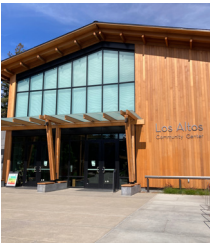
Heavy timber construction
