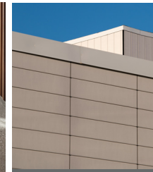
Pre-cast concrete panels
