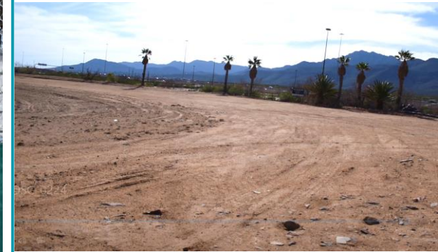
Cohen Stadium Demolition
