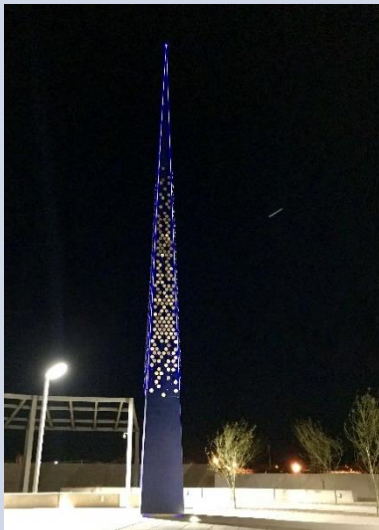
Evening view of installation of Torre de las Flores
