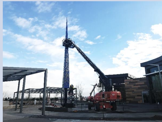
Installation of Torre de las Flores at Northgate
