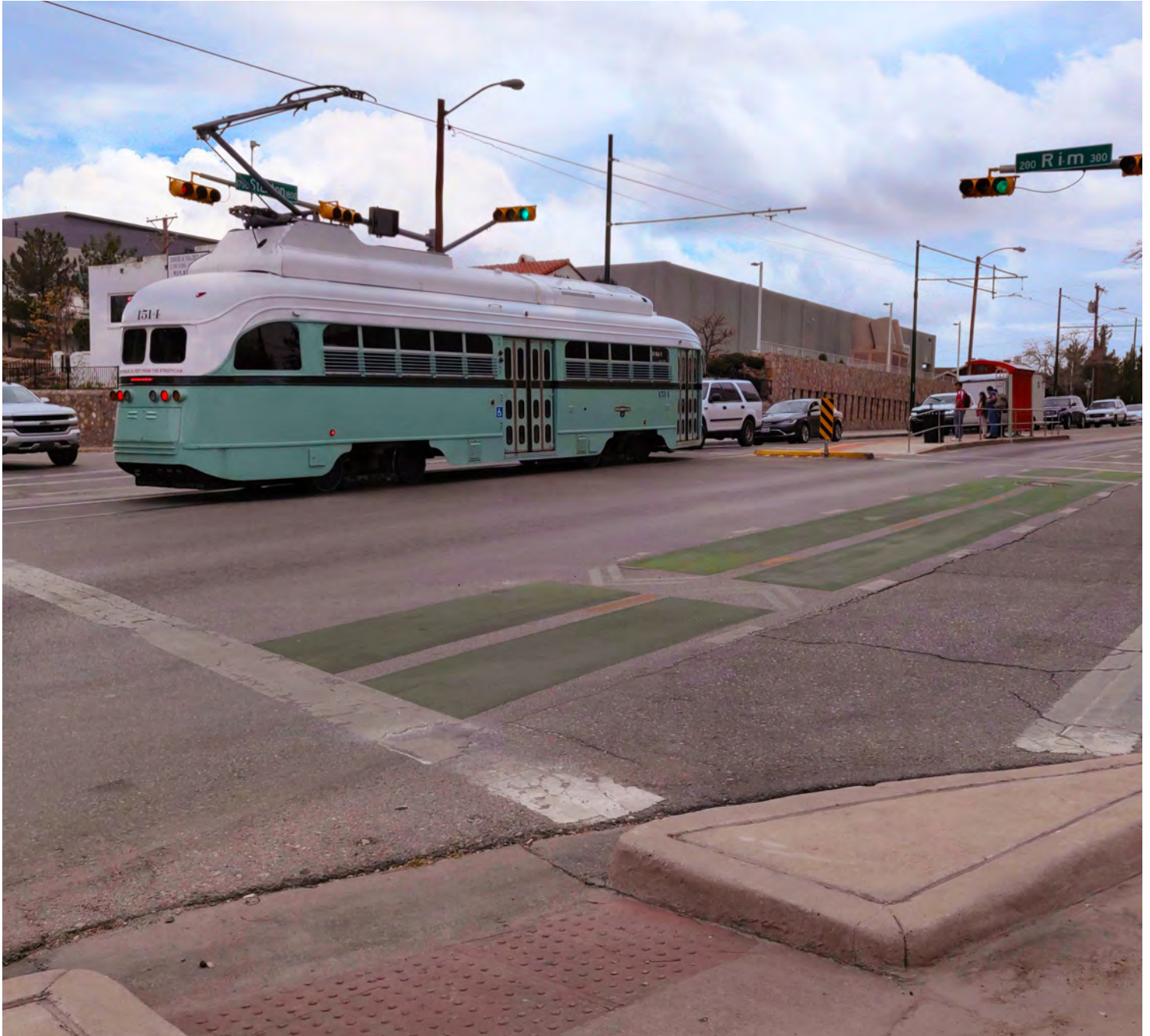
Stanton Street accommodates the needs of all road users, including transit riders of the street car, cyclists within the protected cycle track with dedicated bike signals, leading-pedestrian interval signal phases, and automotive travel lanes.
