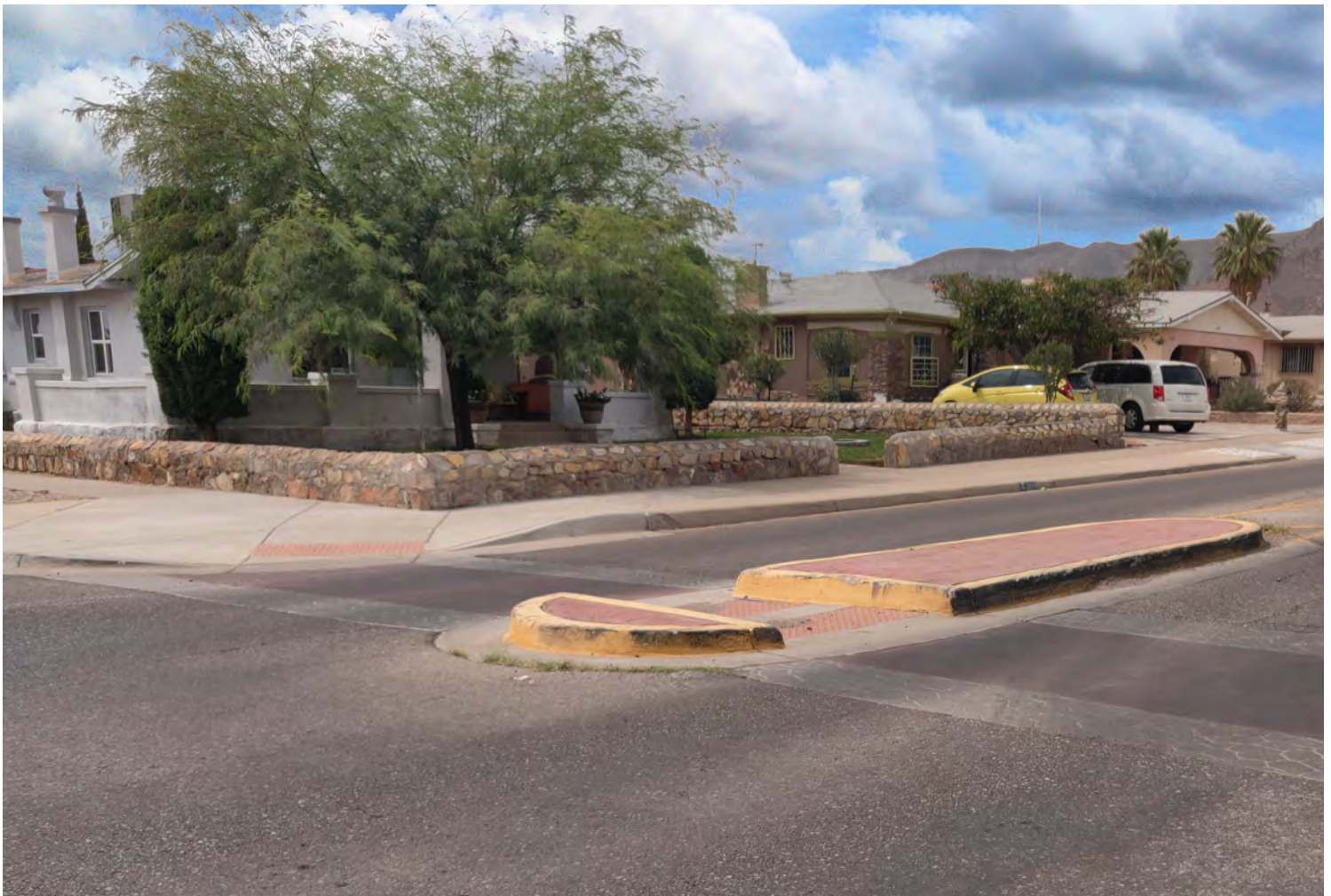
Concrete splitter islands are a complete street design element that reduce the width of a travel lane to promote reduced vehicle speeds; This design also provides a pedestrian refuge within the concrete curb. Textured crosswalk elements promote slower vehicle speeds and colored concrete or painted asphalt alerts drivers to increased pedestrian activity.
