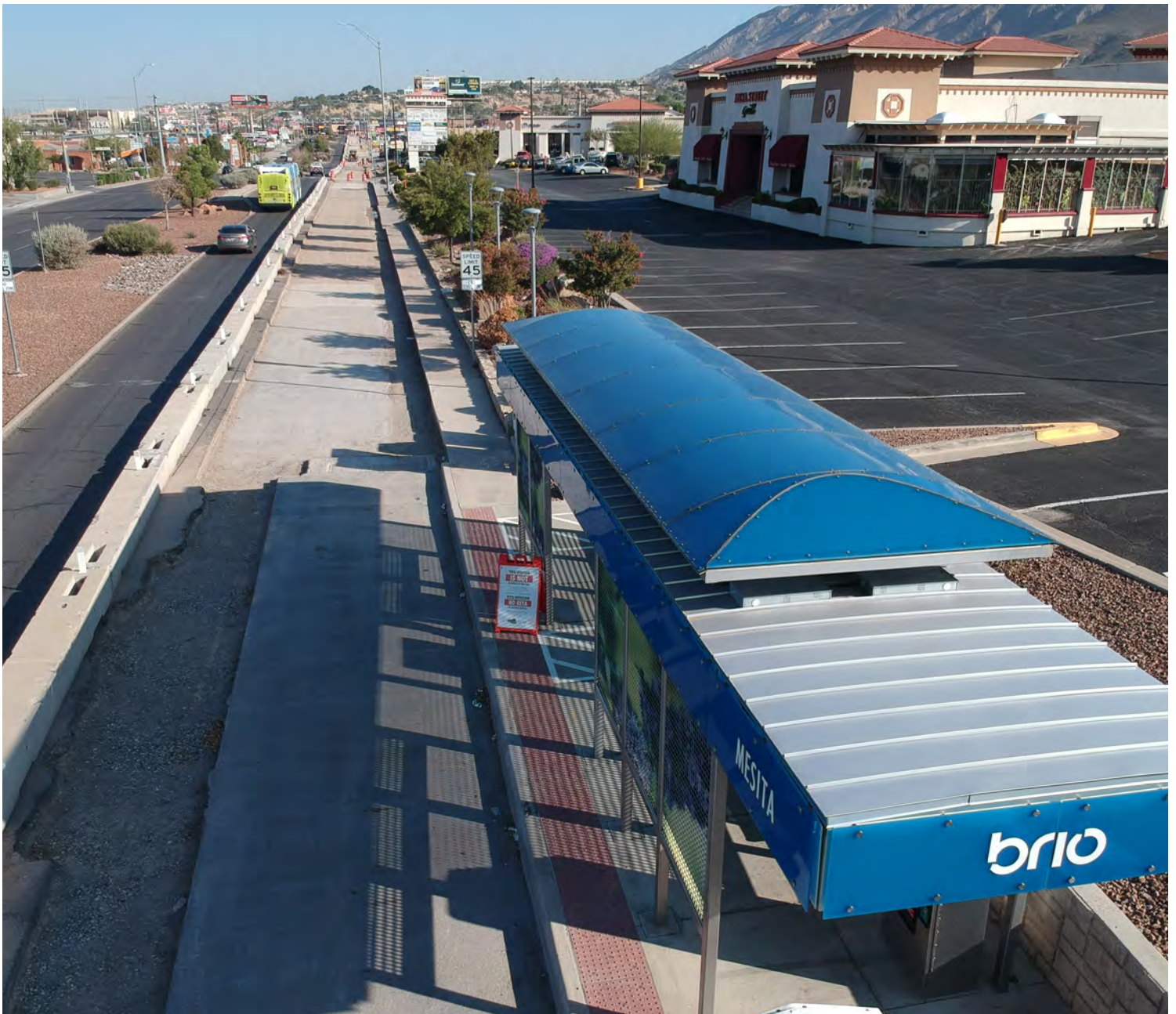
Out of service Brio station due to Mesa Street reconstruction. Close coordination between the City and other project sponsors, such as TxDOT, could lead to expedited construction immediately near transit stops to reduce out of service time.
