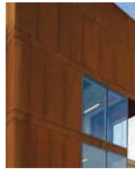
Weathering steel (Corten)
